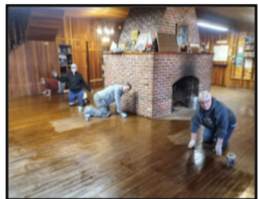
Volunteers refinishing lodge floor
